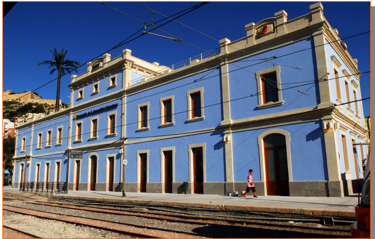
Alicante La Marina station
